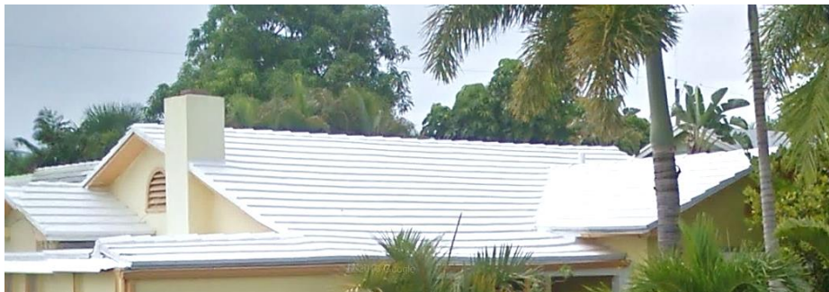
Existing Roof Flat White Concrete Tile
